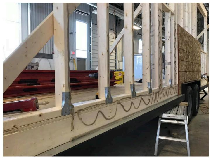
Simpson ties hold studs to the flooring sleepers. The Sill plate is fastened through sleepers and trailer frame. Sheeting is glued to rim joists and studs.
