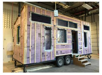
Window flashing installed, rigid insulation on the exterior and then strapped. Dupont flex wrap used around windows to create a window pan that protects against wood rot and moisture. Double pan for added protection.
