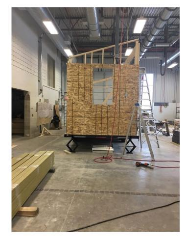
The framing is complete and the house is ready for plumbing and electrical rough-in.
