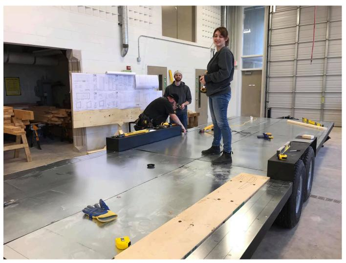
Sheet metal is attached to the trailer to avoid moisture from hitting the underside of the home.
