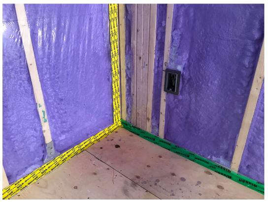
V Barrier is taped in all lap joints and floor intersections.
