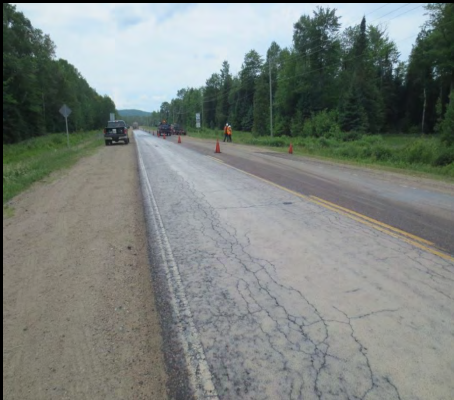
Cracks are partially sealed
